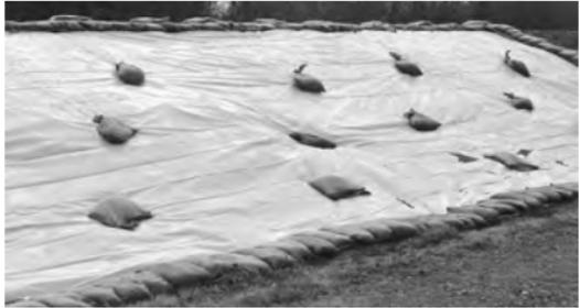
Plastic sheeting is laid out flat on the slope, sandbags are placed around the perimeter with additional bags placed randomly for weight. If the slope is steep, wooden stakes can be driven into the ground just above the area to be protected. The stakes are 4 feet apart with a 1-foot stagger. The plastic is secured to the stakes with tie-down buttons or small round rocks (see Figure 13).
