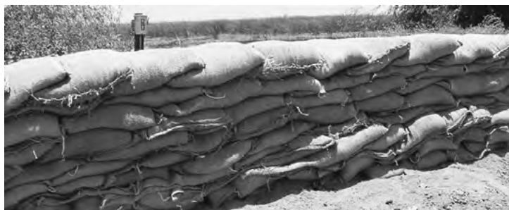
Sandbag Wall Construction
